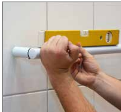
Simple alignment of the bar. An impact marks the second drilling point.
