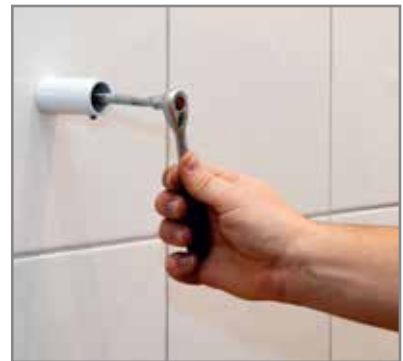
Mount and align the second connection piece.
