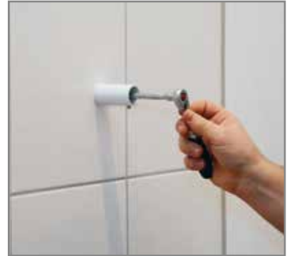
Mount the connection piece to the wall.
