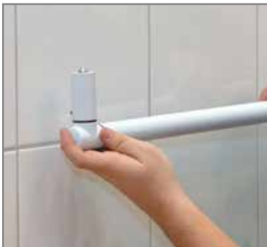
The practical marker (mandrel) helps you to mark out.
