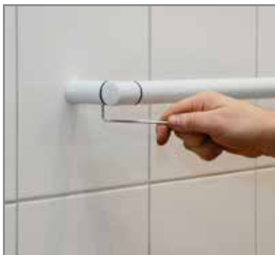
Screw in the threaded pins and tighten.
